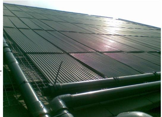
Large EPDM collectors have a positive side effect: since they contain much more water than the boiler, the average salt concentration increases slowly as the water evaporates. With a suitable volume ratio, it is sufficient to fill the system with seawater (4% salinity) before sunrise and to balance only the loss of water with other seawater during the day. By sunset, the salt content has
