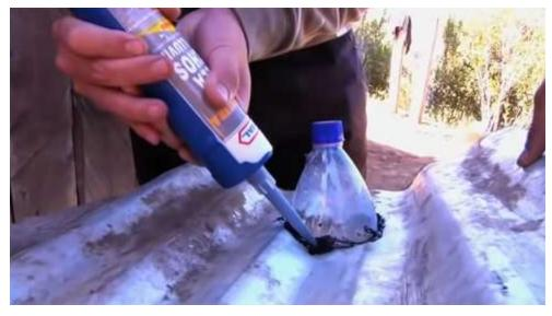
Figure 5. Installation process of Moser lamp (8)
